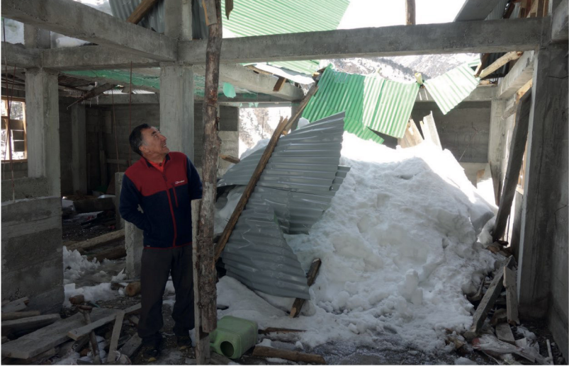
'My hotel is broken.' Winter snow damage at Thangu in Sikkim. ( Mick Fowler )
